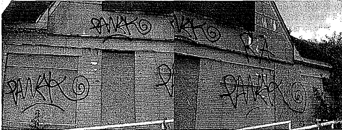
Figure 2: Graffiti at 8094 Delwood St.
