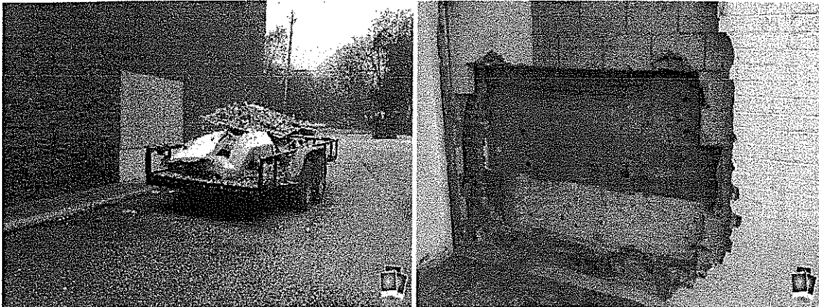
Figure 1: Vehicle attempted to break into store by driving into it.
