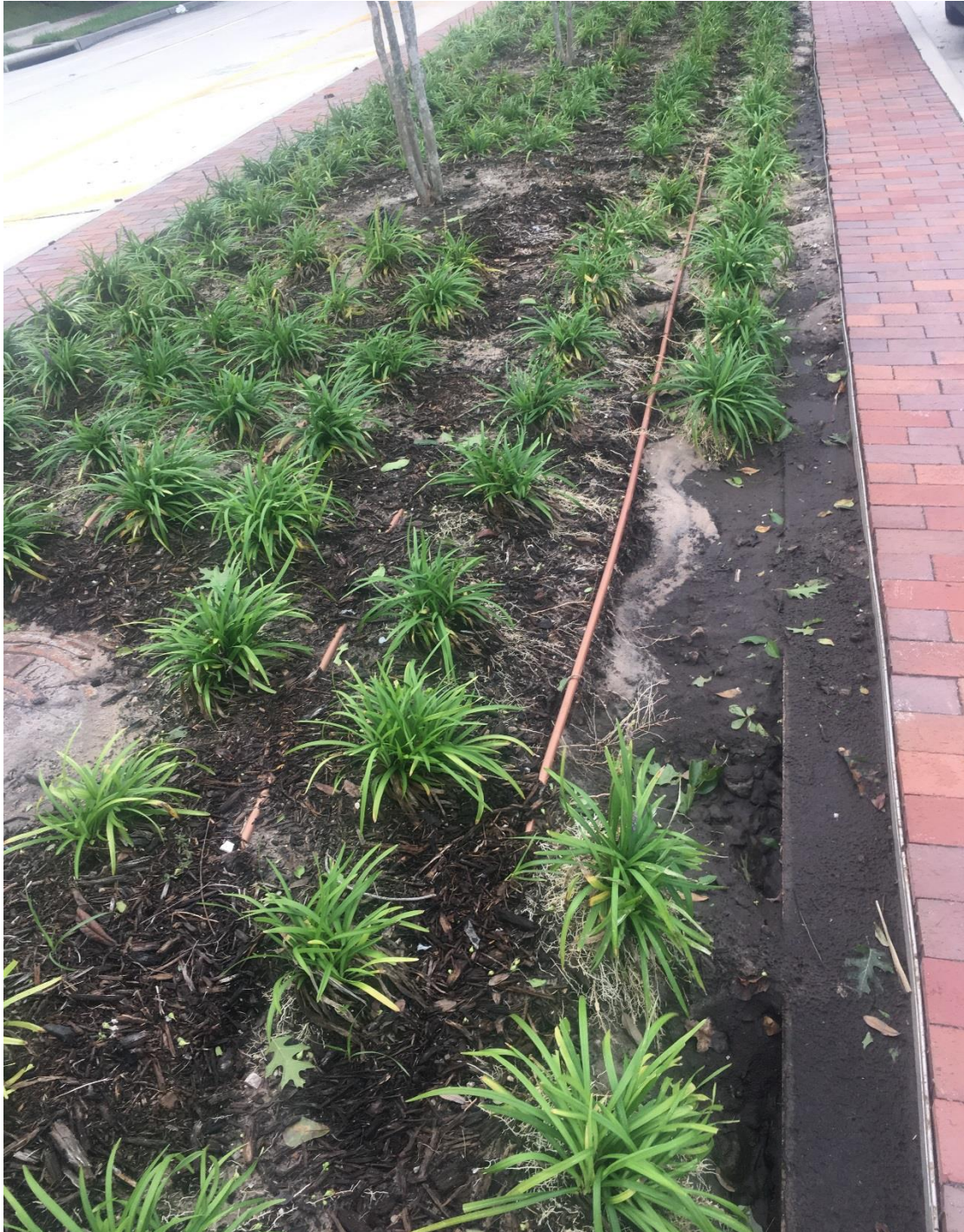
Planting soil and mulch got washed away and the plants were de rooted on a few locations. Replacement of planting mix and mulch is required as soon as possible.
