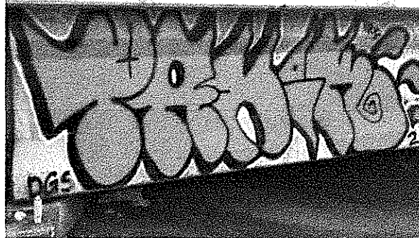
Figure 7: Officer found graffiti on the northbound feeder at Sims Bayou.
